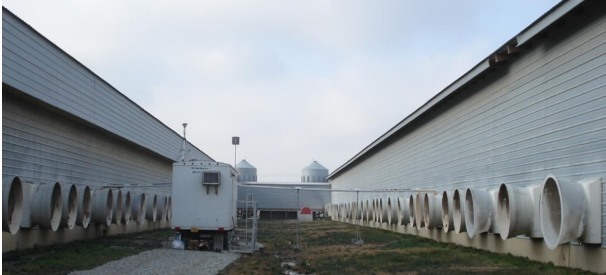
Figure 1. Poultry house ventilation system.
