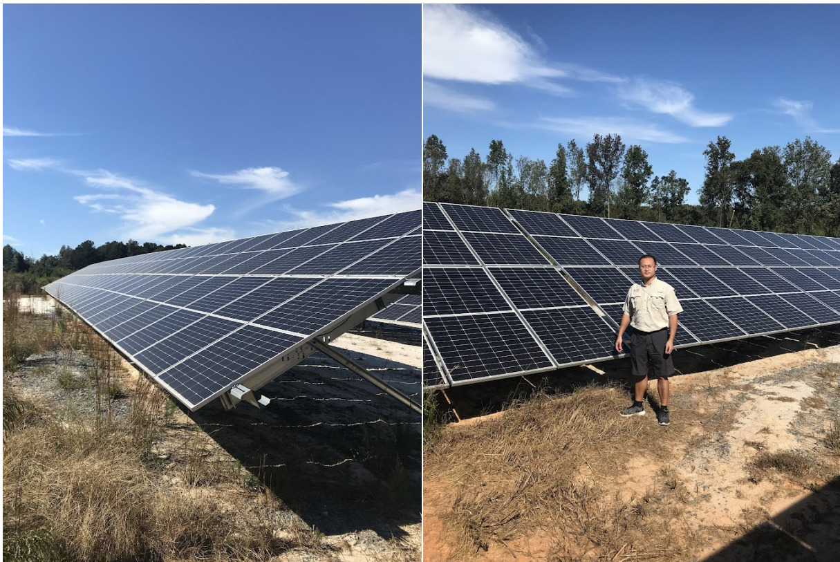
Figure 1. A ground mounted solar power system with panels on concrete floor (photo credit: Lilong Chai).
