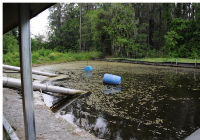
Fig. 2. Inlet piping from irrigation ponds. Note the blue barrels that are keeping the ends of the pipe from sitting on the bottom of the pond.
