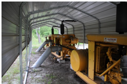
Fig. 5. Diesel powered prime movers for irrigation pumps.
